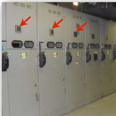
Fig. 1: IR Windows mounted in switchgear
