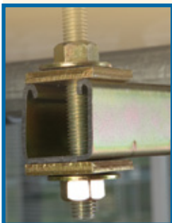
Standard method using nuts and washers
