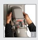
Push the handles up, the plug is fully drawn into the receptacle.
